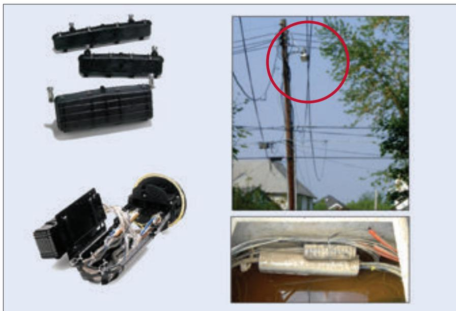
Figure 3.18 – Various splitter enclosures
