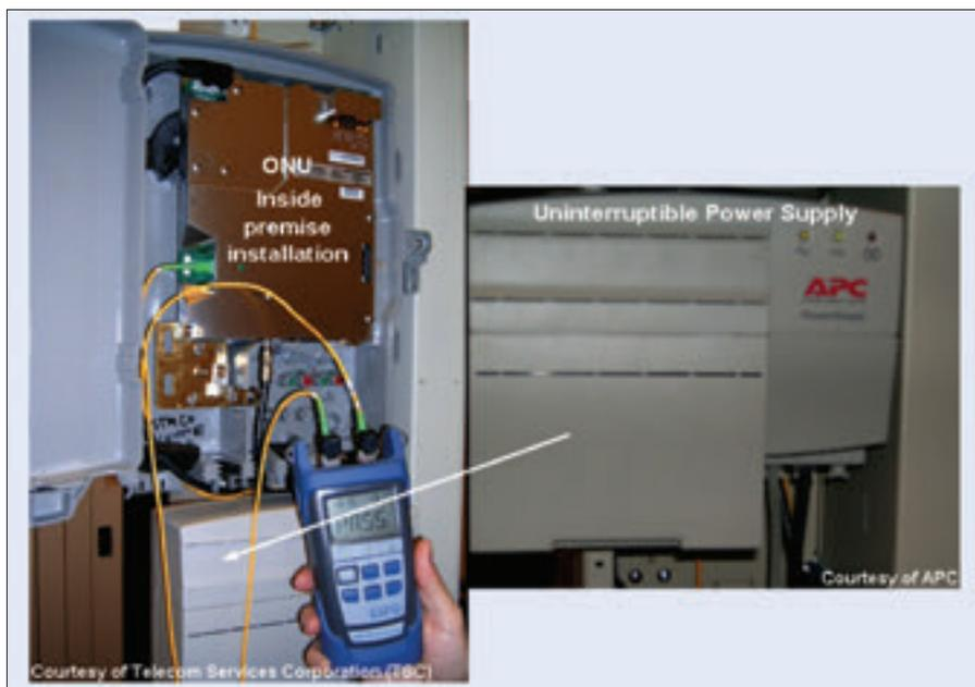
Figure 3.5 – Example of a PON power supply with battery backup
