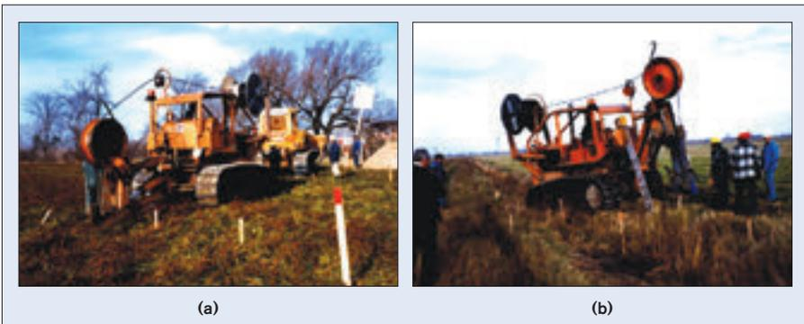
Figure 4.7 – Example of buried cable installation
