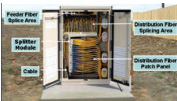
Figure 3.17 – A typical splitter enclosure
