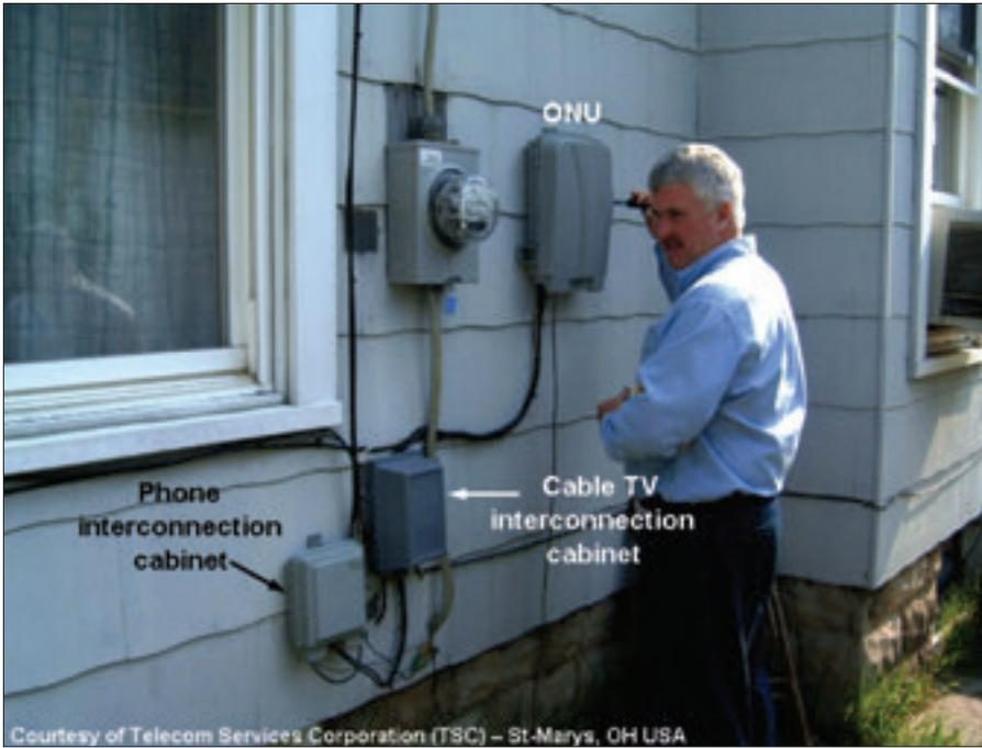
Figure 4.14 – Typical ONT installation completed at the subscriber premises shown in Figure 4.14
