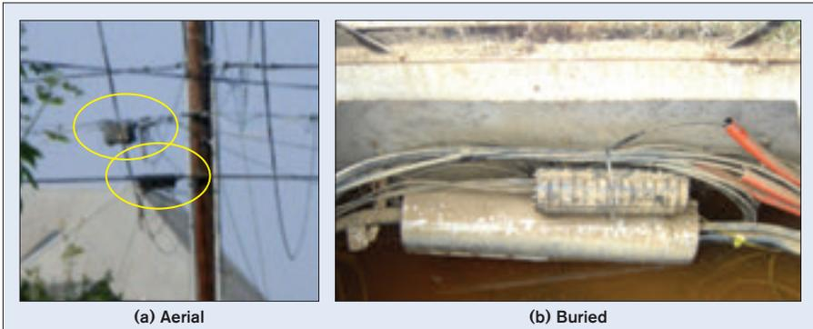
Figure 4.8 – Examples of splice enclosure installation
