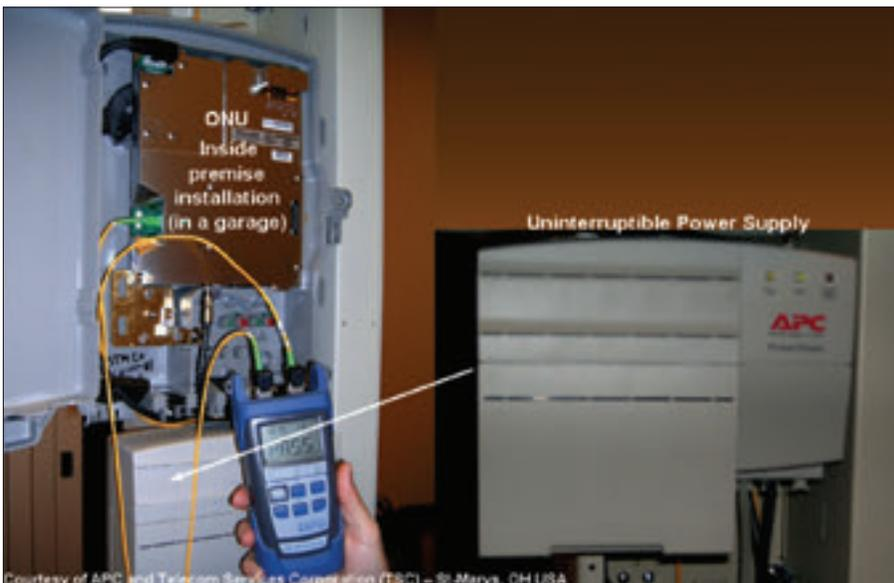
Figure 4.15 – Typical ONU inside-premises installation
