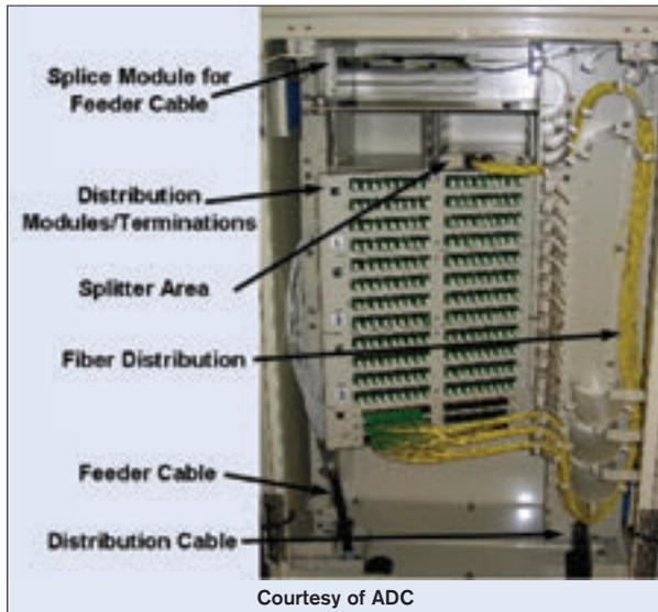
Figure 4.1 -- Typical fiber distribution hub (FDH)
