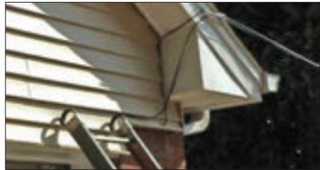
(b) Drop cable installed at the premises
