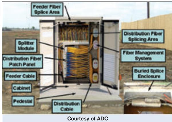
Figure 4.4 – Example of an FDH with buried cable splice enclosure
