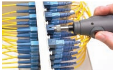
Figure 18 – Patch panel inspection
