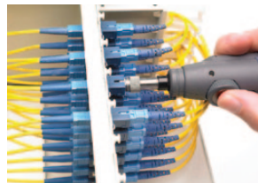
Figure 3-2. Patch panel inspection
